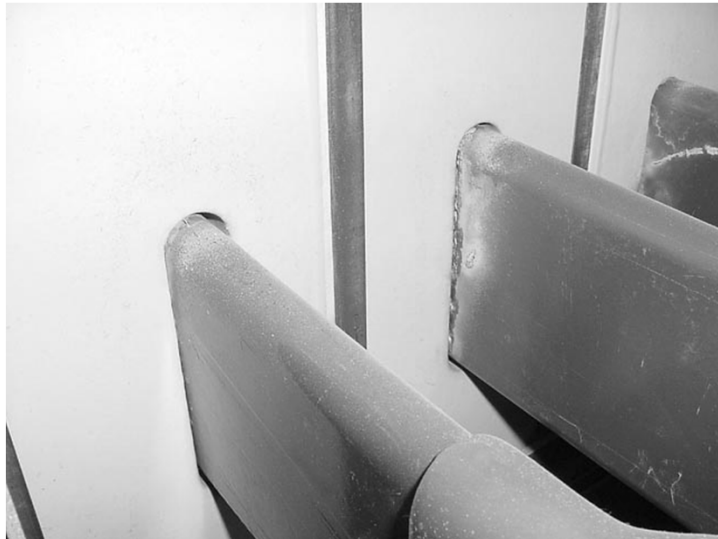
MV Switchgear Buss With CORONA evidence at air-gap between insulating sleeve and cubicle barrier
